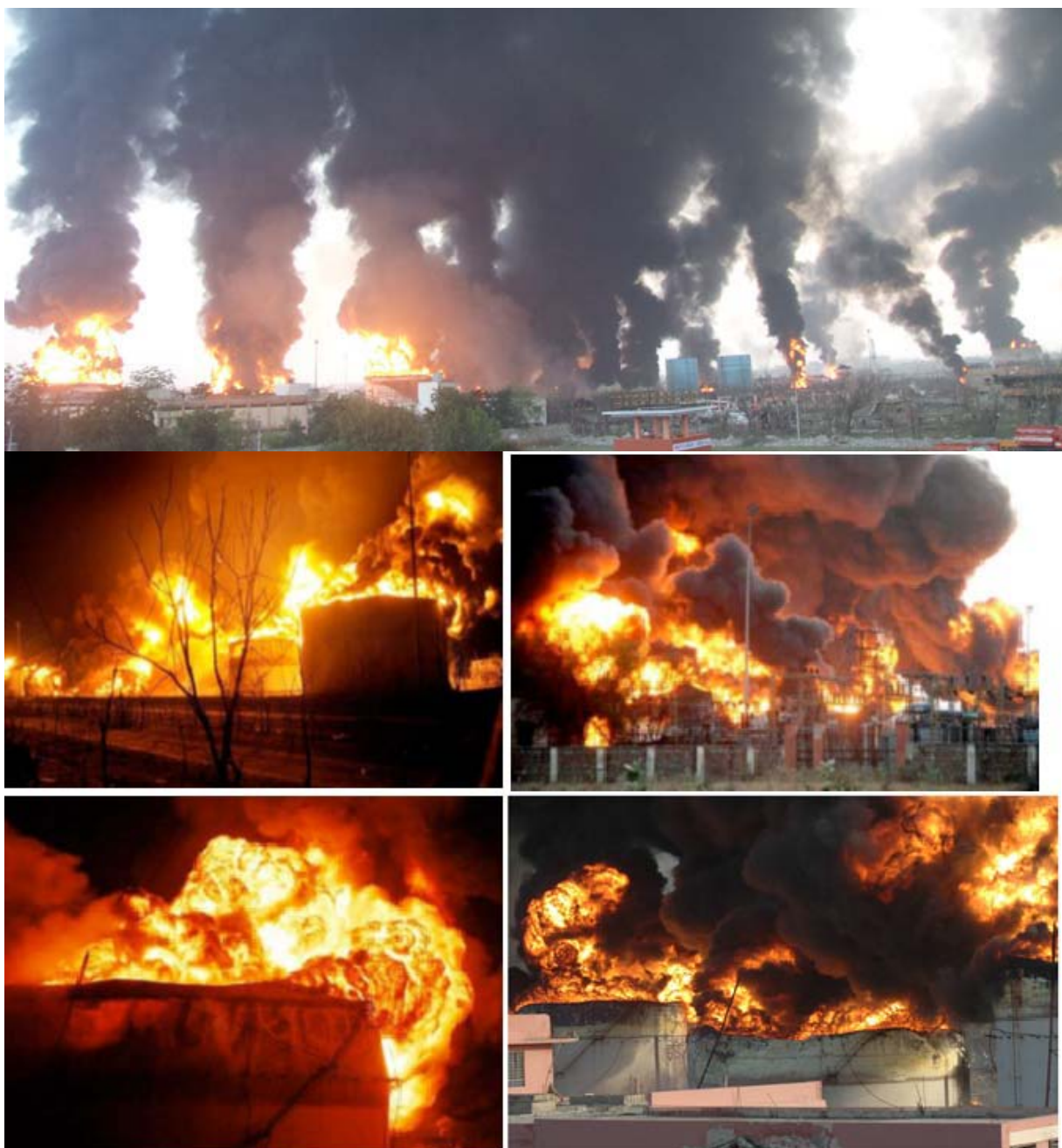
Fig. 5.3 IOCL Jaipur tank fire during the incident (MoPNG, 2010, Roy, 2011)
