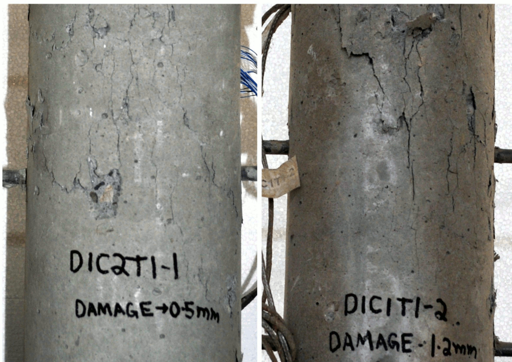
Fig. 3.16: Cracks induced in damage cycle
