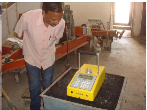
(f) Checking degree of compaction of DBM
