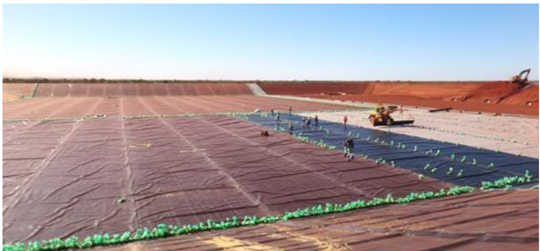
Fig.7 Construction of a tailings dam with lining in Perth (Cape Crushing, 2013)
