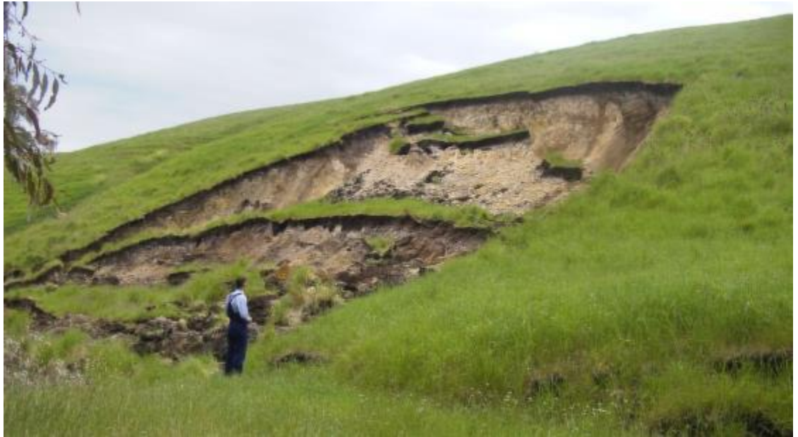
Fig.3 Example of rotational sliding in an embankment
