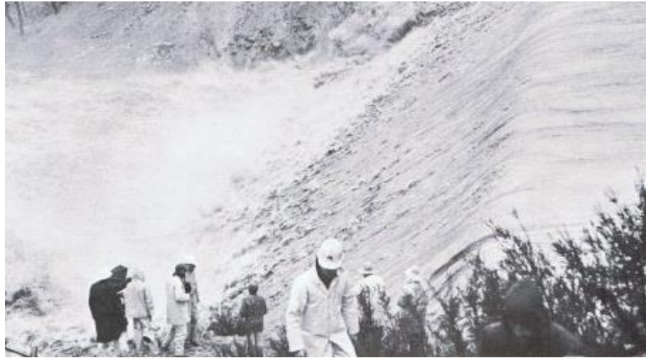
Fig.4 Example of an embankment overtopping (EHA, 2008)
