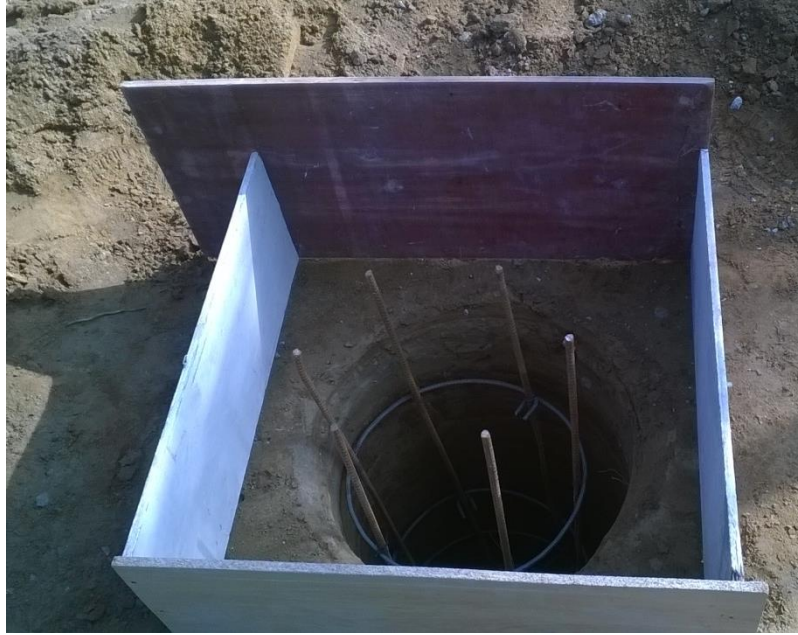
Figure 4-2 Vertical and Transverse reinforcement in Pile stem
