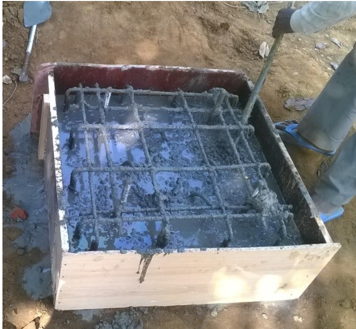
Figure 4-4 Showing construction process
