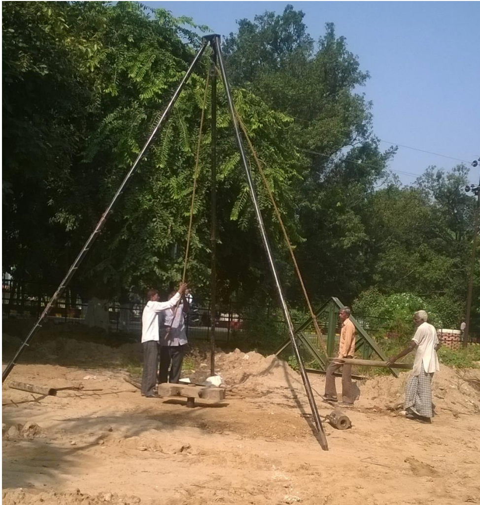
Figure 3-1 Performing Standard Penetration Test at the site
