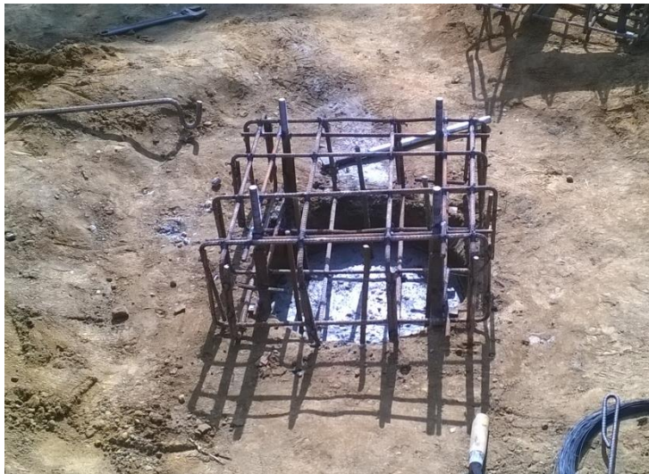
Figure 4-3 Showing the reinforcement in the pile cap
