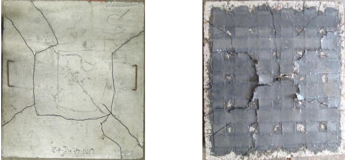
Figure 5.16 (a) Cracks on top face of USG-70 (b) Cracks on bottom face of USG-70
