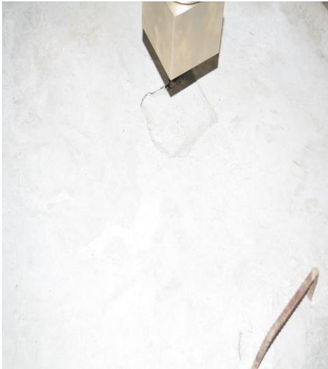
Figure 5.8 (a) Punching on top face
