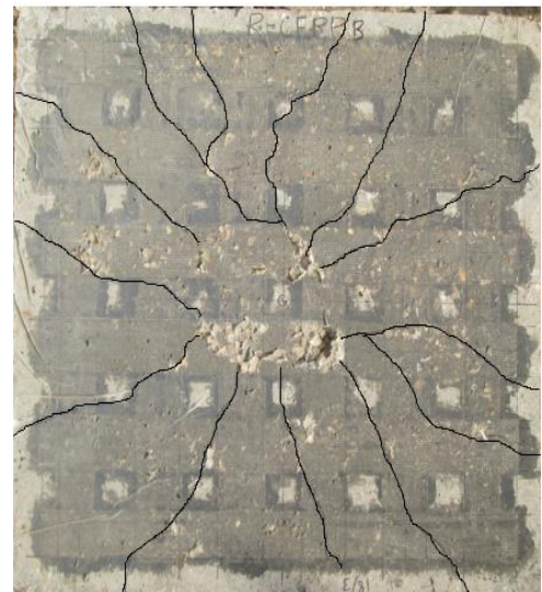
(b) Cracks on bottom face of RSC-70
