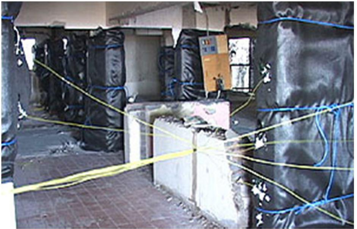
Fig. 2.12. Columns loaded with charge wrapped around by geo-textile.
