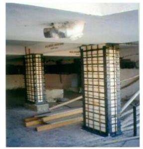
Fig.2-7- Construction Technique for Steel Jacketing
