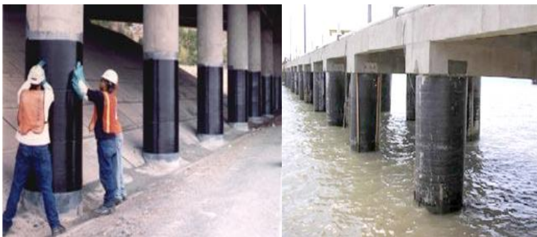
Figure 6.8 Carbon fiber reinforced polymer jacketing of bridge bent
