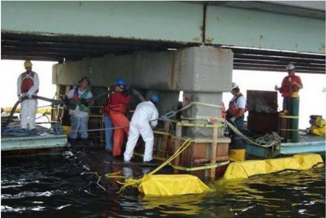
Figure 6.1 Reinforced concrete jacketing of bridge bent
