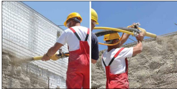
Figure 1.4: Shotcreting of wall and slab panels
