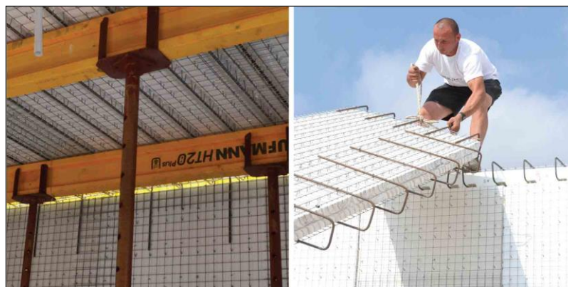
Figure 1.3: Placing of slab panels on top of wall panels
