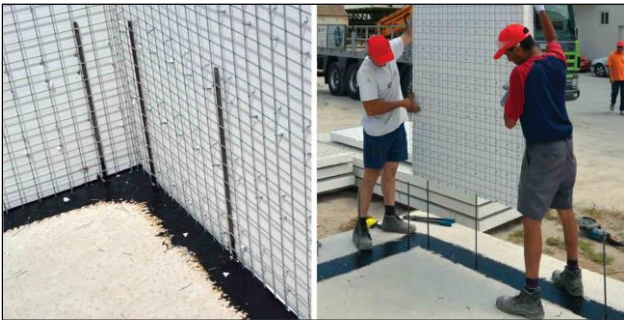
Figure 1.2: Erection of EPS wall panel on top of foundation
