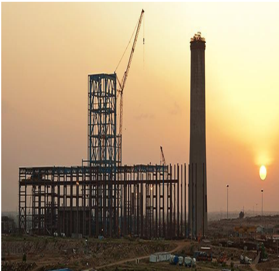
Figure 3.1 NTPC Gadarwara (Main power house building)
