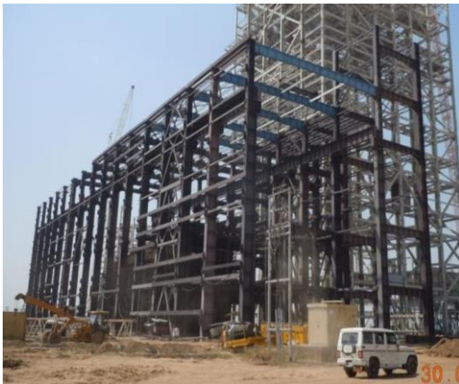
Figure 3.8 Ongoing construction at site
