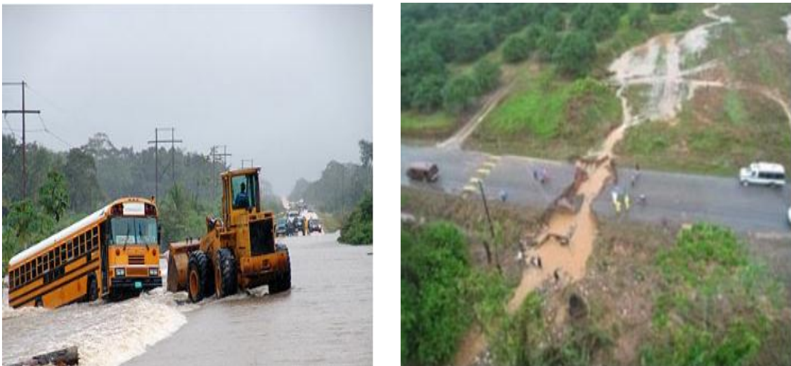
Figure 3.7 Image showing damages caused due to floods
