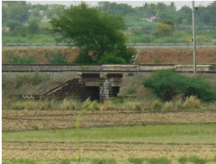
Figure 3.10 Railway bridge opening (water way)
