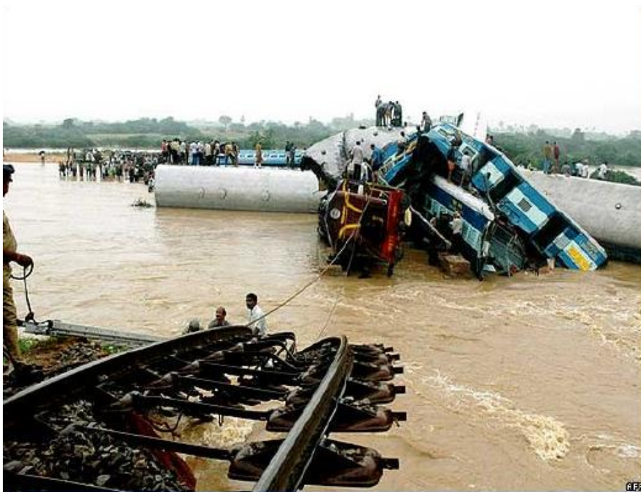
Figure 3.12 Image showing train derailed due to subgrade erosion of embankment
