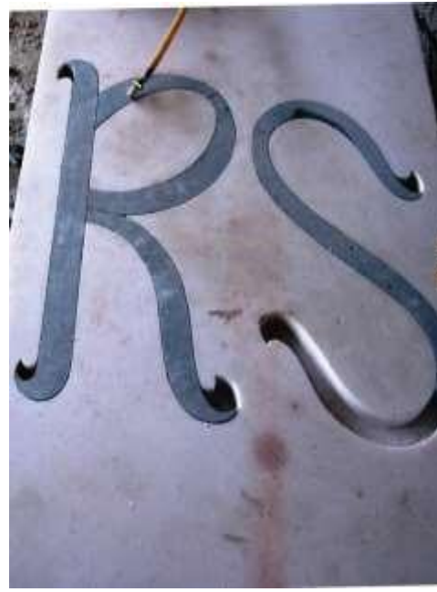
Fig 3.7 Fixing of coloured stone
