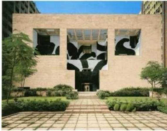
Fig 5.4 British Council Library Front Façade: Tree of Knowledge the British Council HQ in Kasturba Gandhi Marg, New Delhi, designed by Charles Correa, showing the front mural facade by Howard Hodgkin. Completed in 1992, it evokes the shadows cast by a tree and is executed in black stone and white marble tiles.
