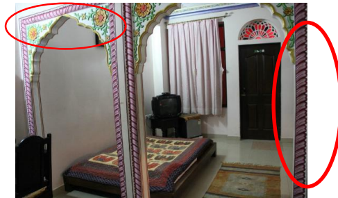
Fig 5.28 Painting & Stucco decoration in residential building of Jaipur
