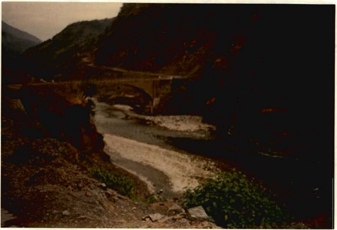
Plate 6.5 Runoff Gauging Site at Yashwant Nagar
