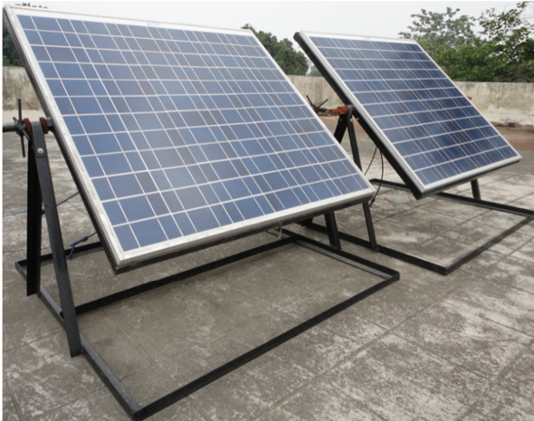
(a) PV Modules
