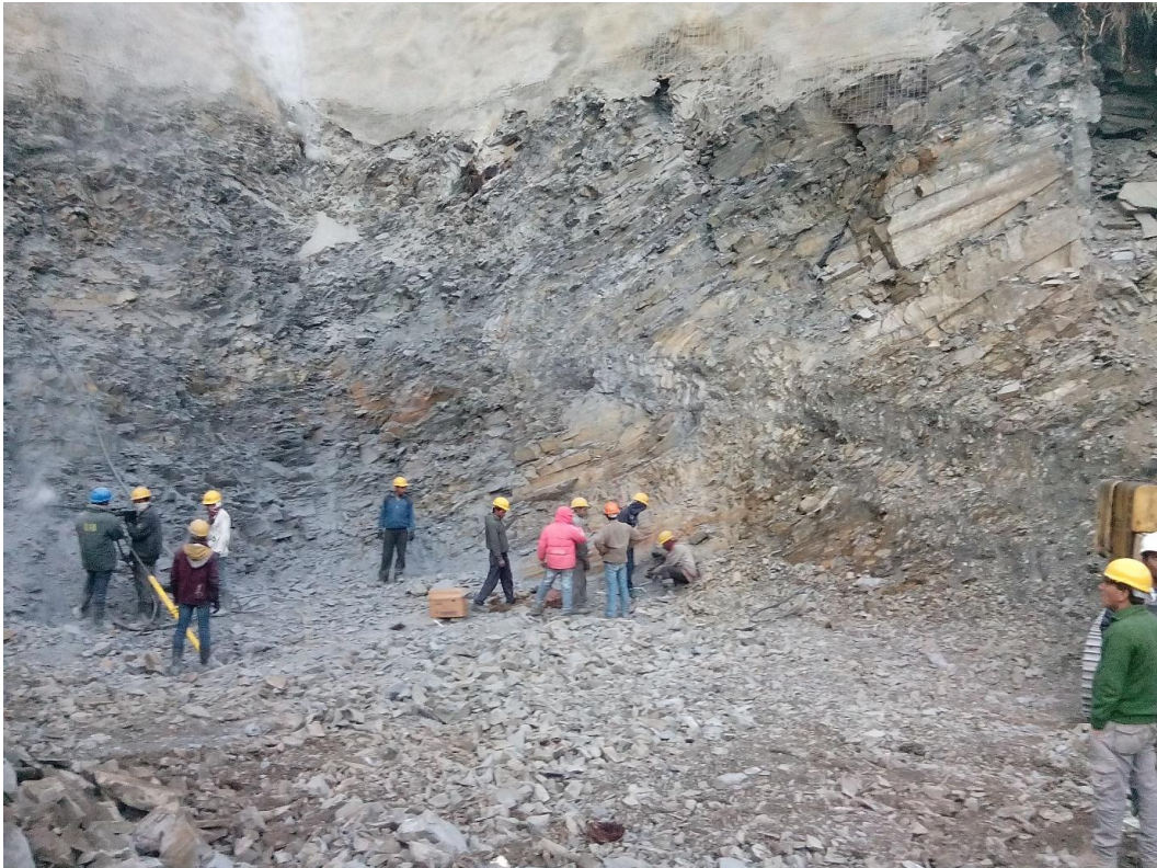
Fig 3.4 Presence of slate just above the drift opening at Hat village
