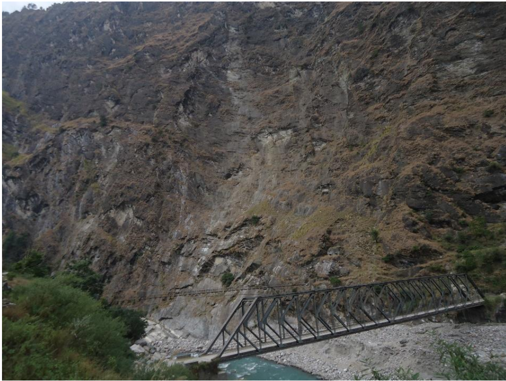
Fig. 8.26 Foliated stained granitic gneissic rocks exposed near Urgam bridge
