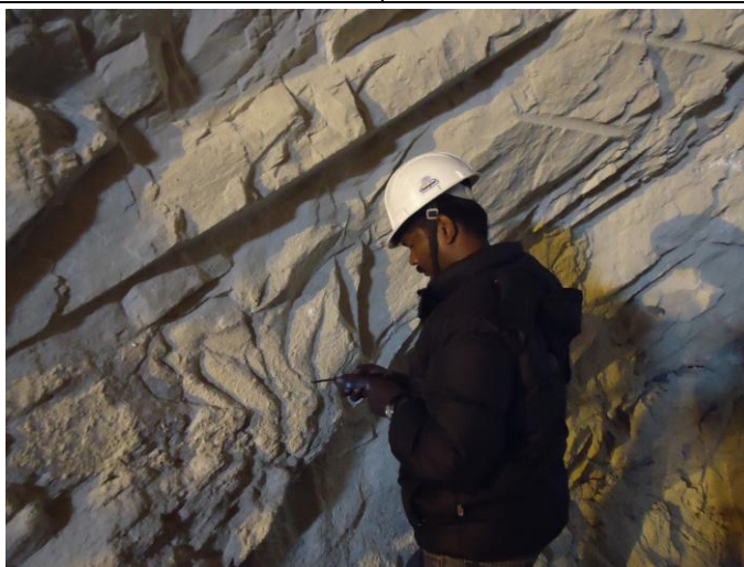
Fig 4.11 Fresh light grey colored quartzite seen in diversion tunnel near dam site
