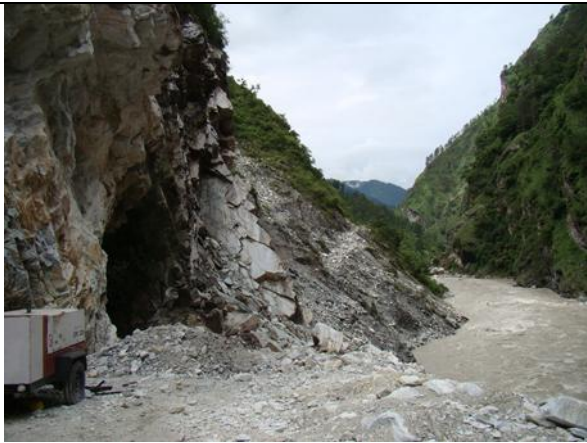
Fig 4.9 Drift-DL-01 on the Left bank at dam site
