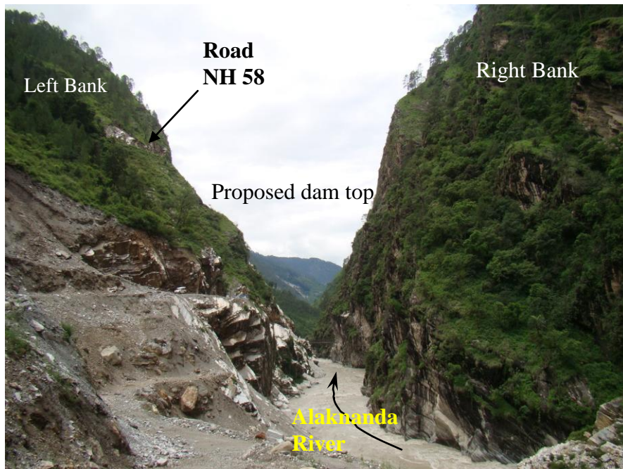
Fig 4.2 Steep narrow gorge of VHEP dam area with massive Garhwal quartzites
