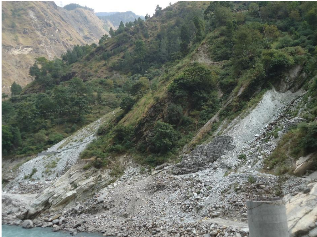
Fig 8.29 Debris and RBM material present along section L6
