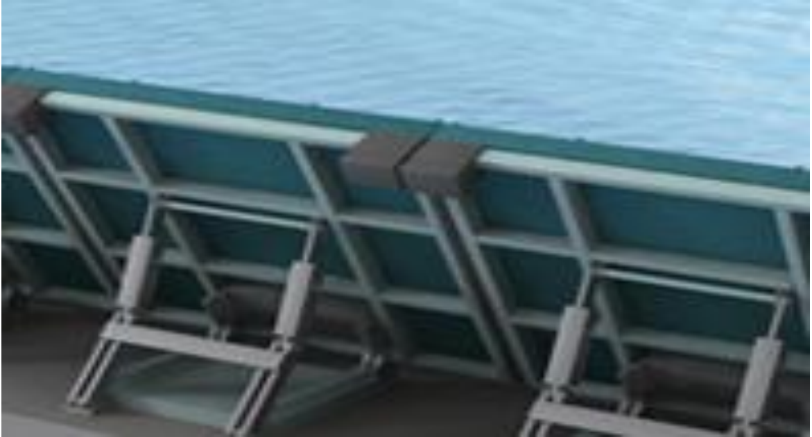
Figure 3.8 Folding Fusegate in operation
