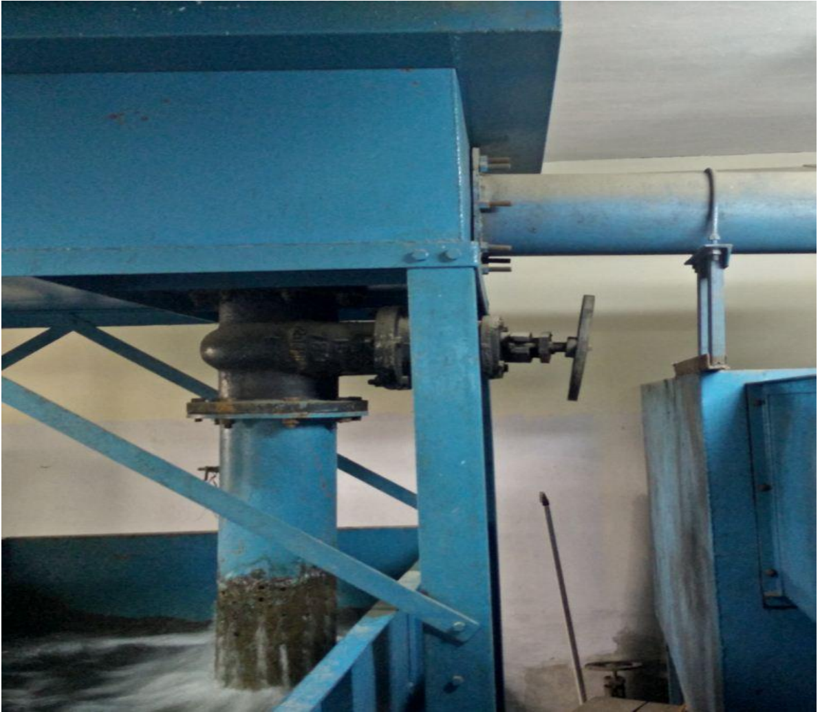
Figure 6.2 Discharge control mechanism
