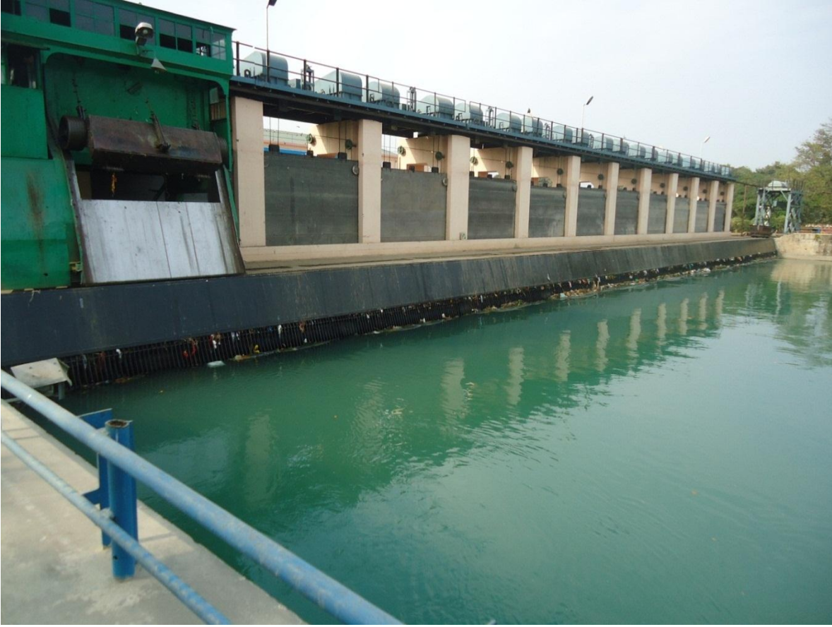
Fig 4.11:-Trashrack at Pathri Powerhouse
