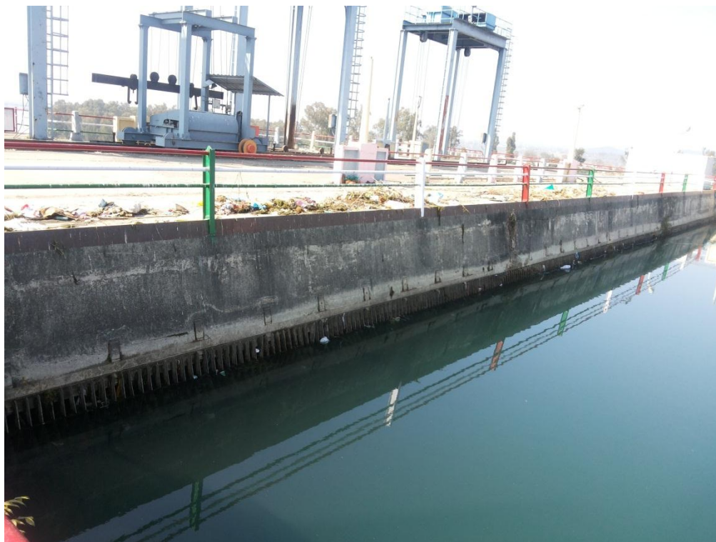
Fig 4.16-:Trashrack At Dhalipur
