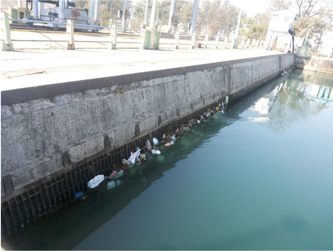
Fig 4.14:-Trashrack At Dhakrani
