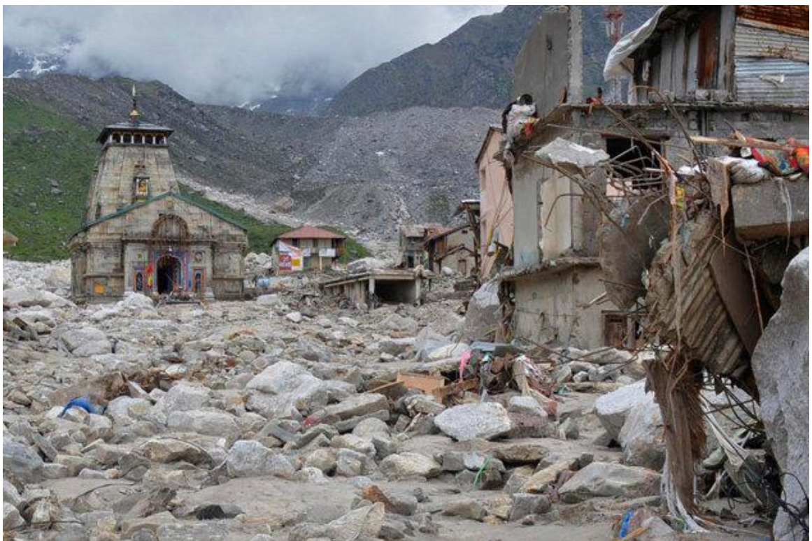
Figure 2.2: Damage caused by cloudburst induced flash flood near Kedarnath temple
