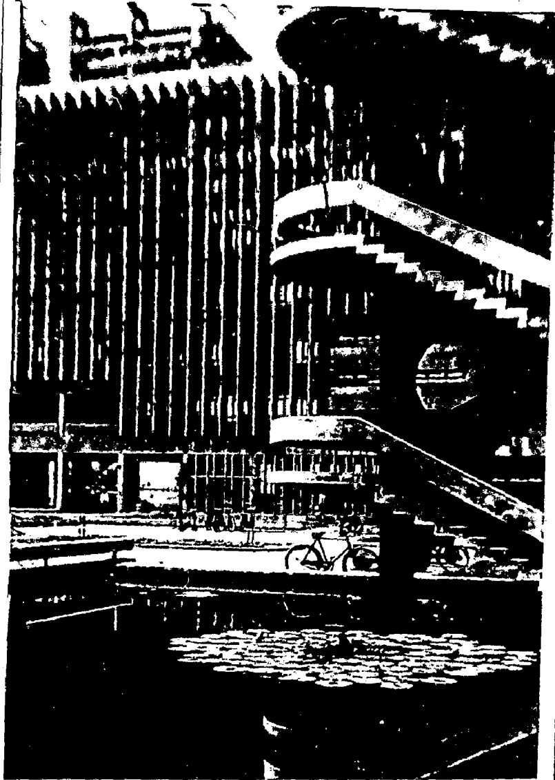
IIT DELHI, multi story academic building which dominates the center of the campus — all departments are linked together in this complex.
