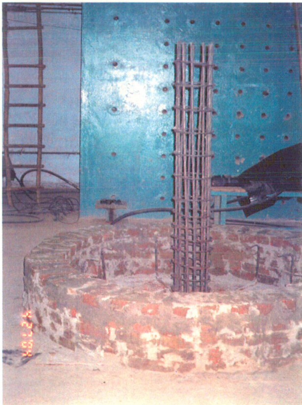
Plate 3.2 Formwork of Model M1 and M2 before Casting
