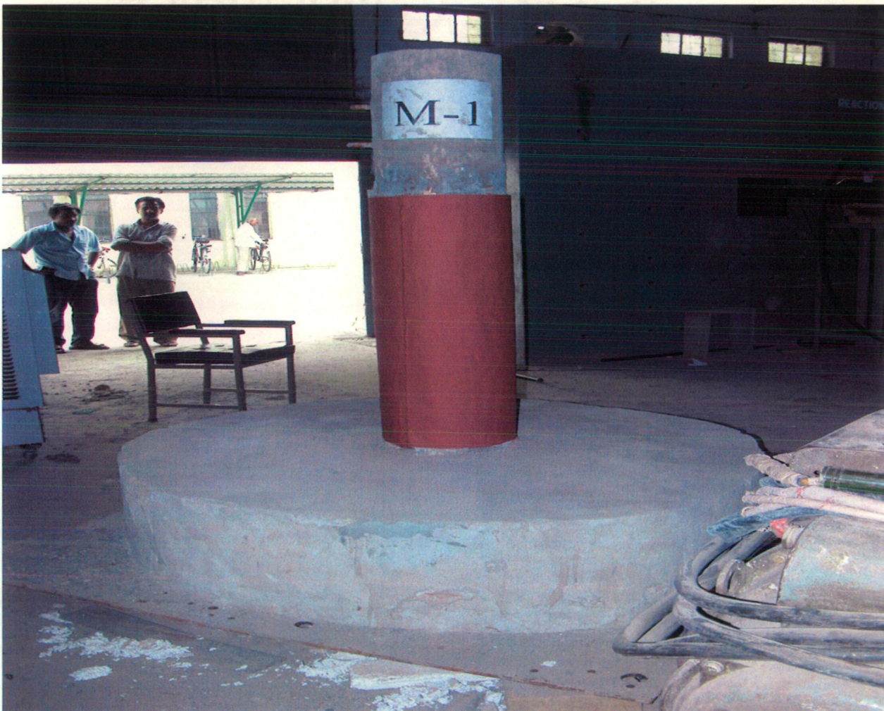
Plate 5.5 Model M1 after Retrofitting with steel jacking
