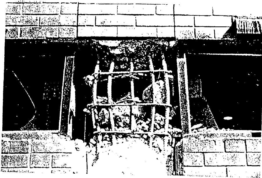
Influence of partial height infill increasing column shear force
