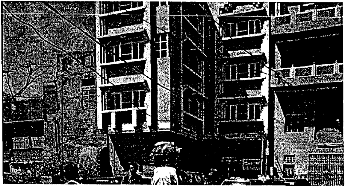
Photograph 8.5: Punjabi tower at Main Chaura Rasta, constructed by demolition of old Haveli. (Feb., 2004)
