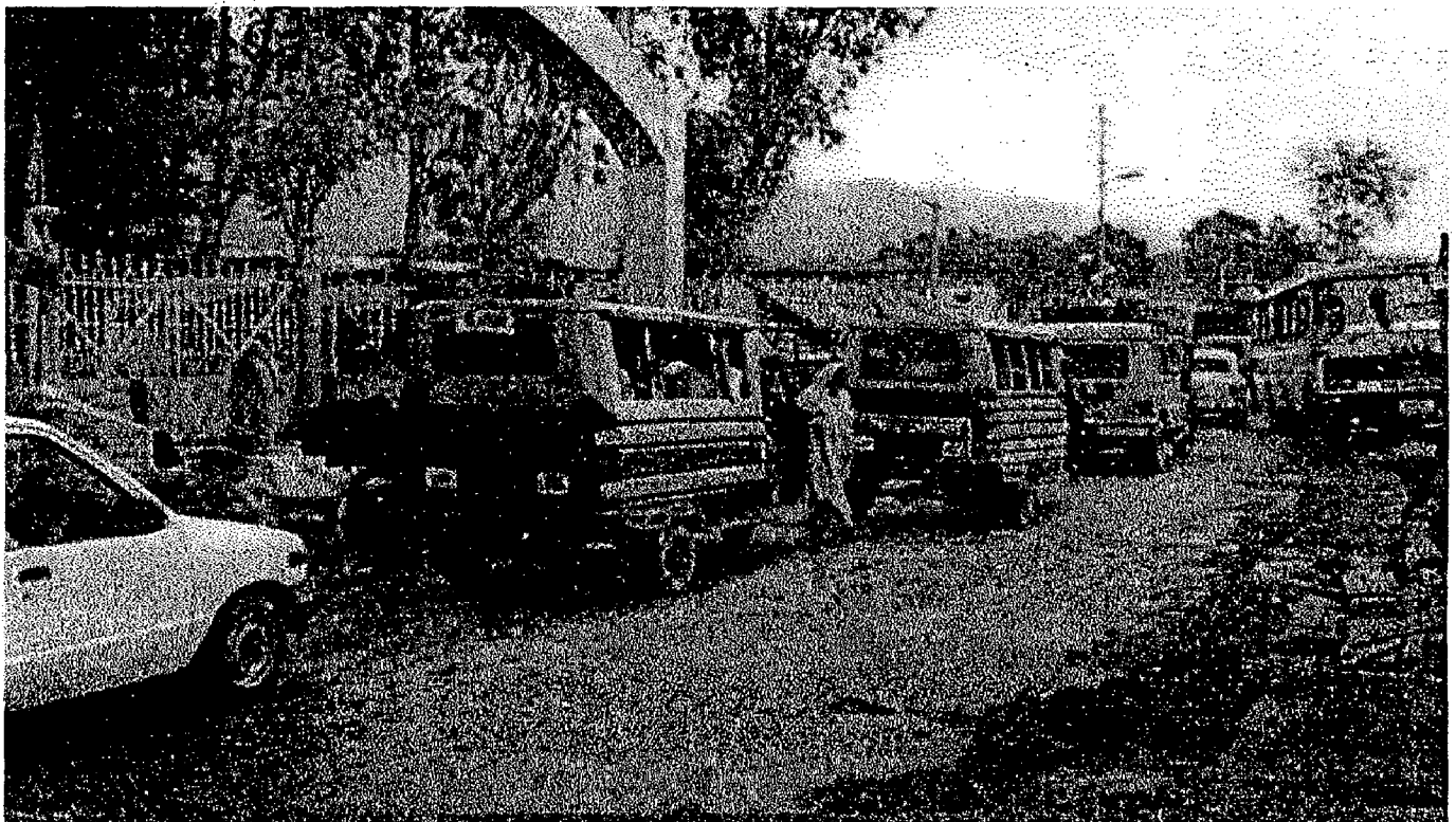
Poor Drainage Condition of the Parking Places
