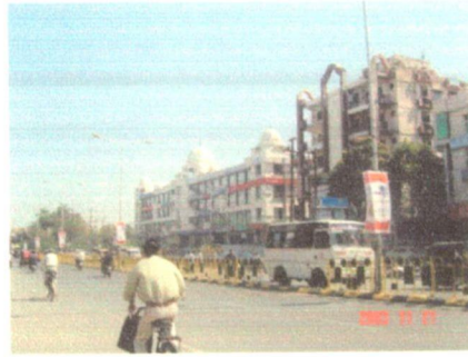
Fig. 5.25 Indraprastha Tower, M.G. Road
