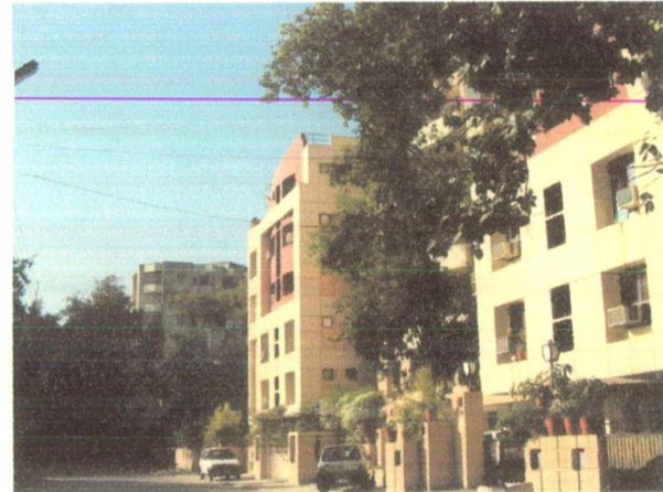
Fig 4.7 Old Palasia, a bungalow converted into flats
