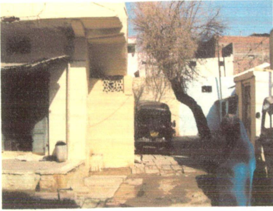
Fig. 5.34 A water connection in Nanda Nagar.
