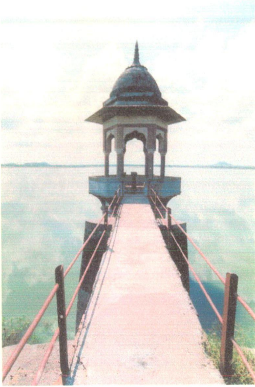
Fig. 5.44 Bilaoli Filter Tank
