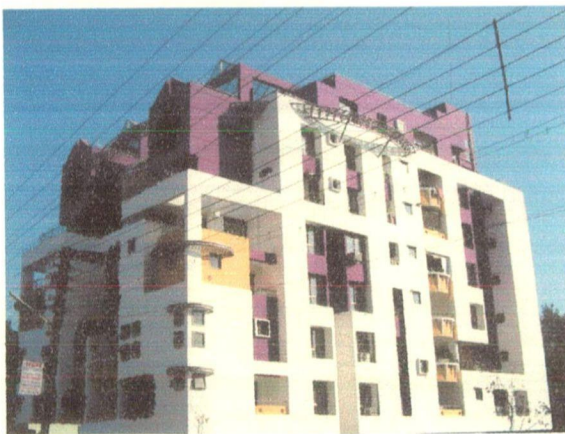
Fig.5.30 : An apartment housing in Old Palasia Area
