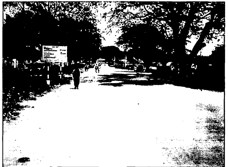
ILLUSTRATION 5: VIEW OF THE DODDABALLAPURA - DEVANAHALLI STATE HIGHWAY PASSING THROUGH THE DODDABALLAPURA TOWN
