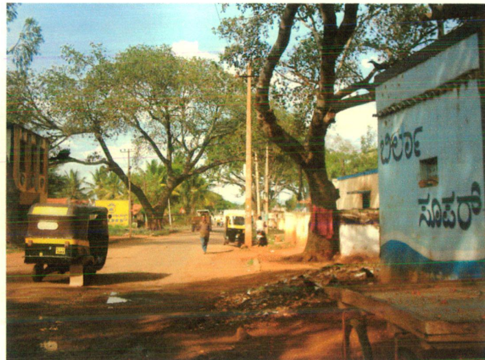
ILLUSTRATION 17: VIEW OF ROAD CONDITION WITHIN THE DODDABLLAPURA TOWN
