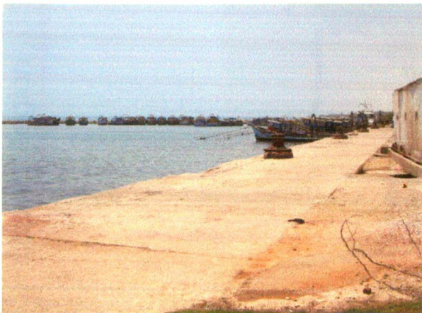
(vii) Landing Center at Mandapam
