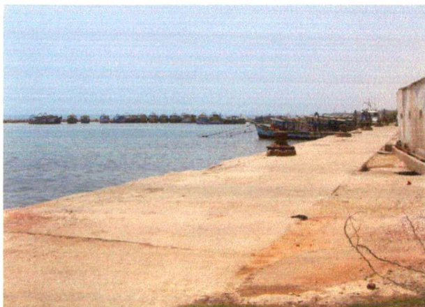
(vii) Landing Center at Mandapam
