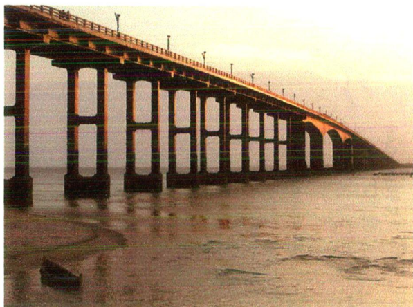
(vi) The Pamban Bridge *
