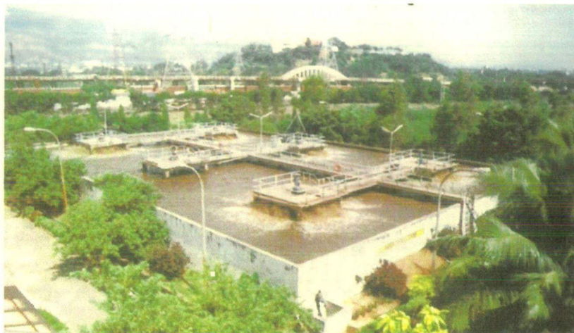
Fig 5.7: Existing sewerage treatment plant : Block 1
