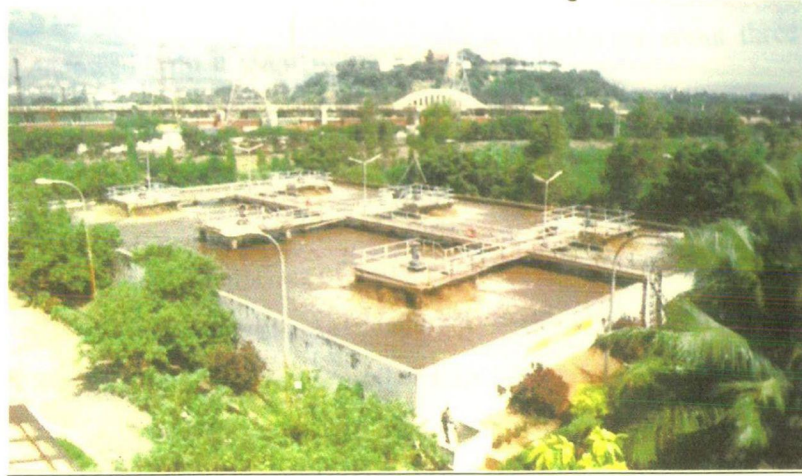
Fig 5.7: Existing sewerage treatment plant : Block 1
