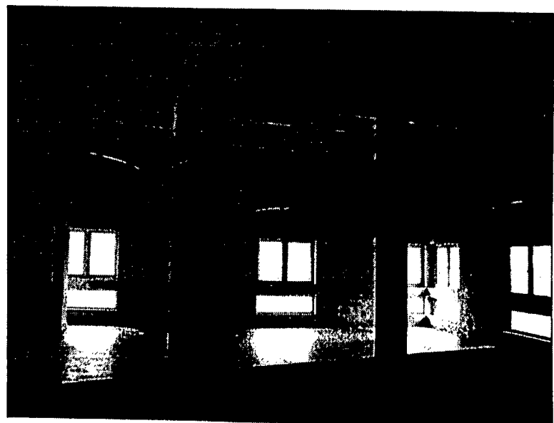
Fig (6.6f): low Height windows for Daylighting
