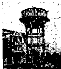
Fig 5.6 m Over Head Tank
