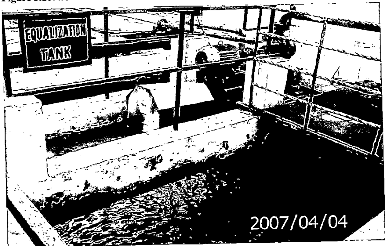
FIGURE 5.11: EQUALIZATION TANK AT OKHALA
