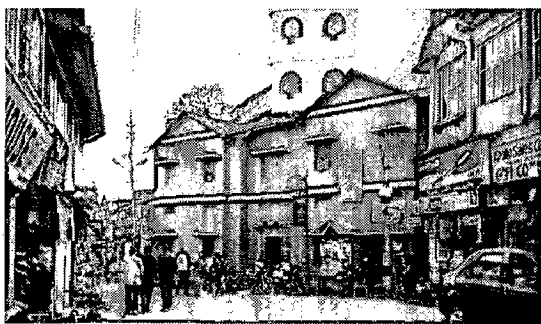
Fig. Police Station – Mussoorie
