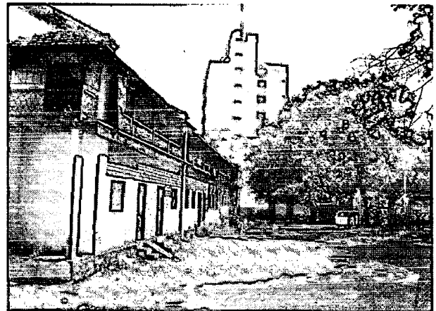
Figure 6.6 Dilapidated structures in Zone A
