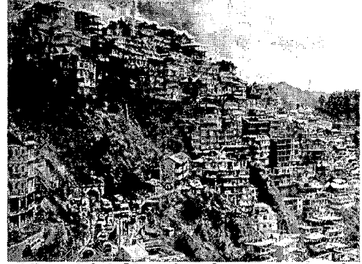
Visual 6.6: Massive Construction in Cemetery without proper Accesses
