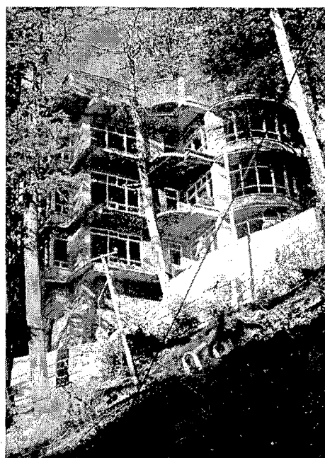
Visual 6.4 :R.C.C. construction threatening green belt in Jakhu Area.
