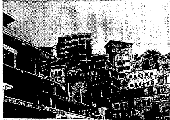
Visual 6.2: Massive Constructions in Jiwanu Colony
