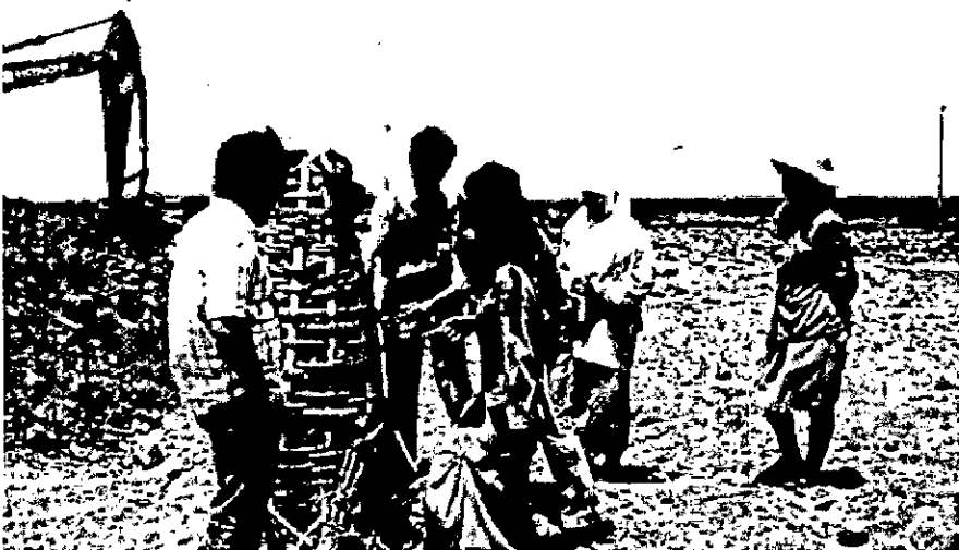
Figure 2.6 Gas venting cage made of bamboo in Indonesia
