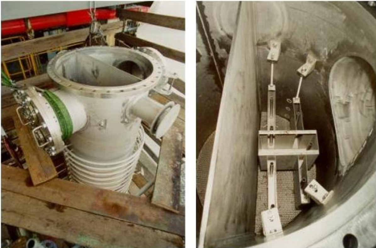
Figure-4: A welding of the divided wall in to the column
