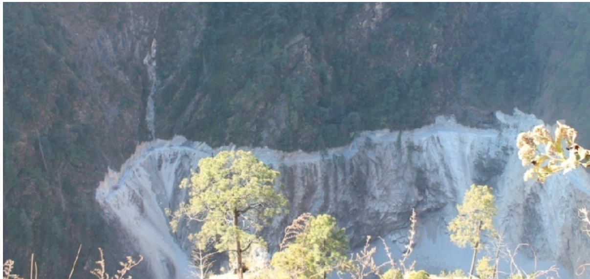
Figure 55: Road construction going on in study area
