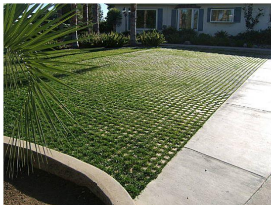
Fig. 5.3 Grass-crete used instead of Paved Concrete or Asphalt
