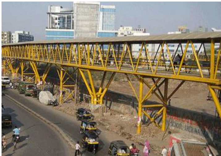
Figure 2.7 Pedestrian skywalk in Mumbai
