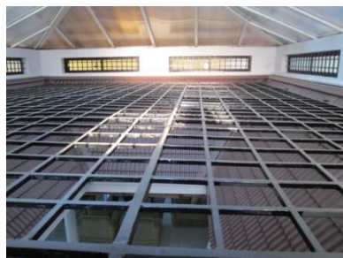
Figure 121: roof of the courtyard has been covered for safety reasons
