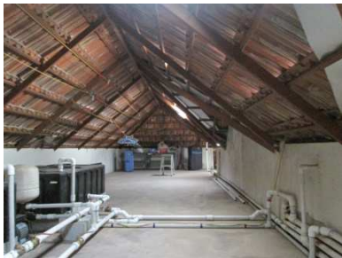
Figure 81: ventilated attic space used as a store
