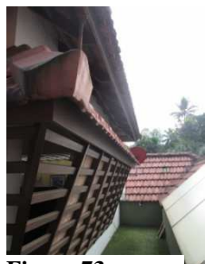
Figure 73: inclined wooden louvers
