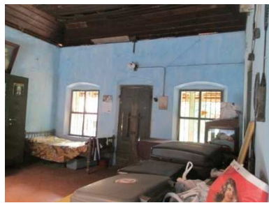
Figure 48: hall near the courtyard
