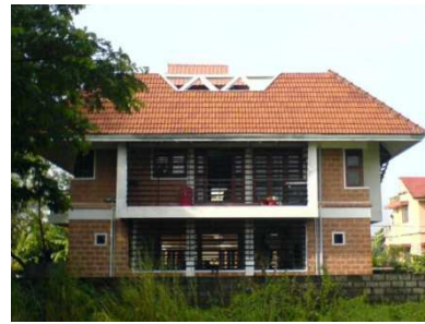
Figure 83: view from the main road
