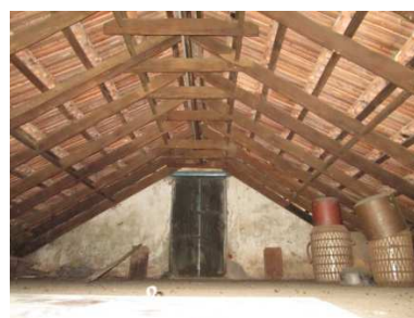
Figure 54: Attic space used as storage & provision for ventilation is given
