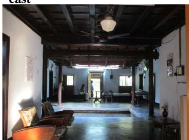
Figure 69: straight aligned openings
