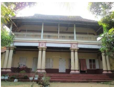
Figure 45: Front verandah & entry to the house
