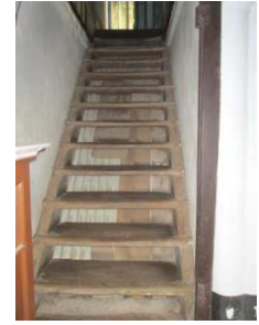
Figure 33: staircase leading to upper floor
