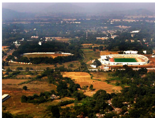
Figure 79 - Aerial view of Ispat Stadium and Biju Patnaik Hockey Stadium in Rourkela
