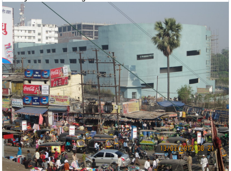
Figure 14 The temporary shops and the visual chaos and aesthetic disorder clearly seen in front of the entry and exit point of the railway station
