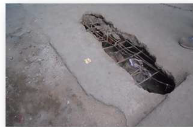
Covering of Open drain
