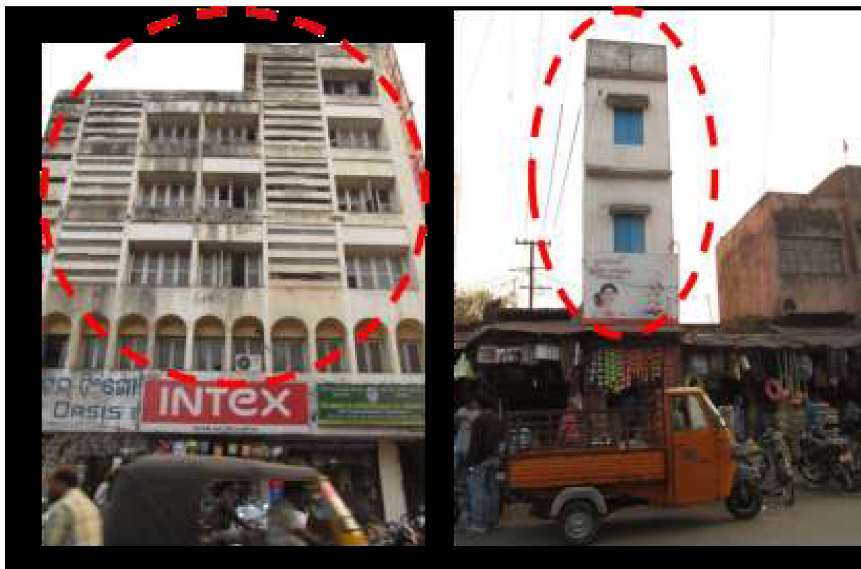
Figure 16 image showing violation of building bylaws
