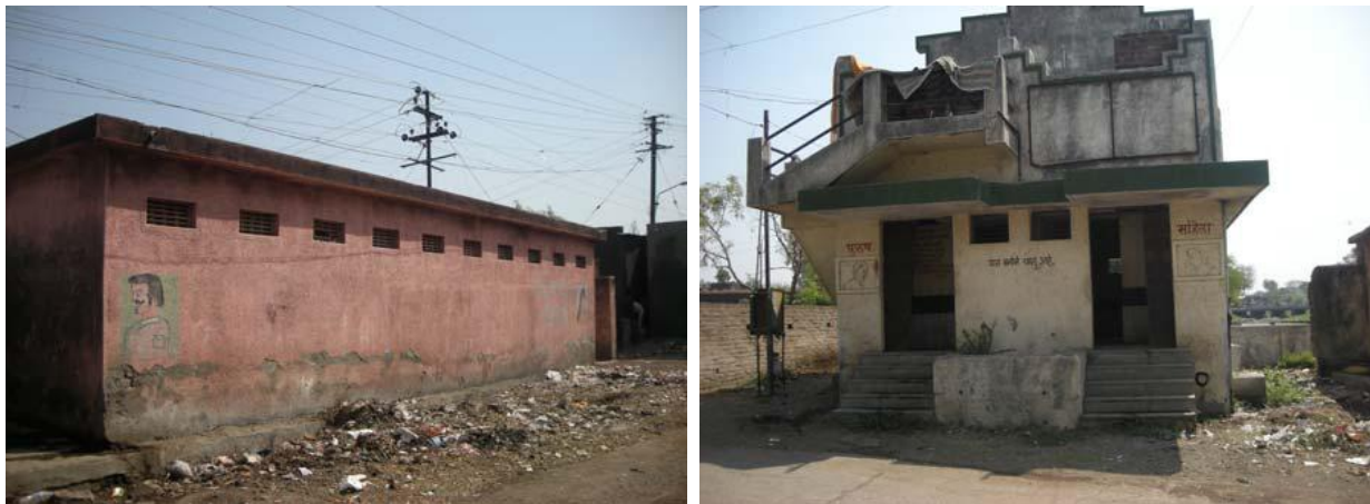
Figure 22- Poorly maintained public toilets
