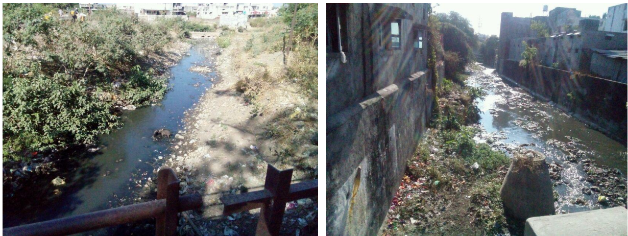
Figure 25- Poor condition of rivulets in the city
