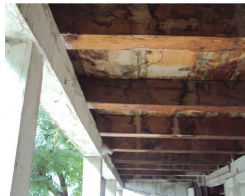
Figure 28: Planks laid over secondary beams
