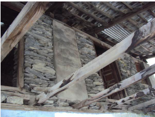
Figure 29: Stones filled in the gap between secondary beams
