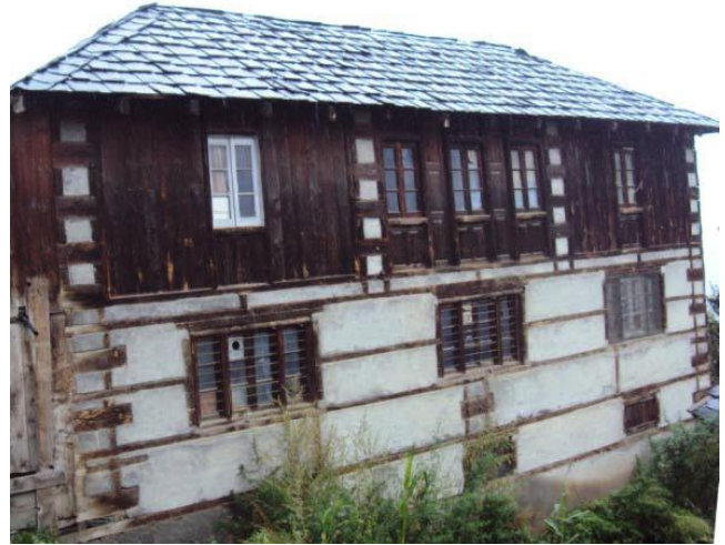
Figure 16: Thathra house in Chamba
