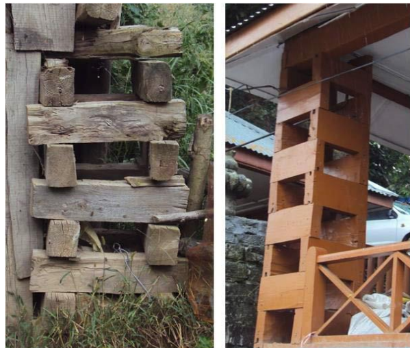
Figure 18: Hollow box-like frame for thathara
