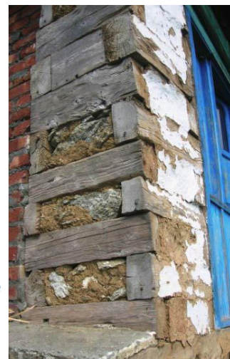
Figure 19: Thathara with stone and planks laid together
