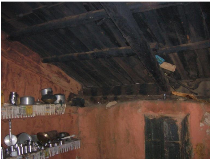
Figure 62: Connection between roof and wall in structure at village Bharmour
