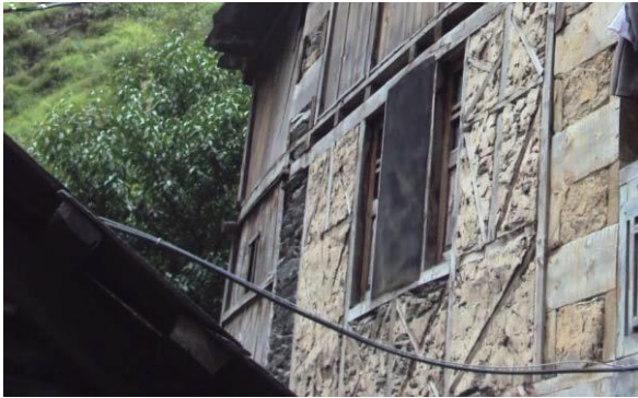
Figure 25: Diagonal bracing of wood in infill wall
