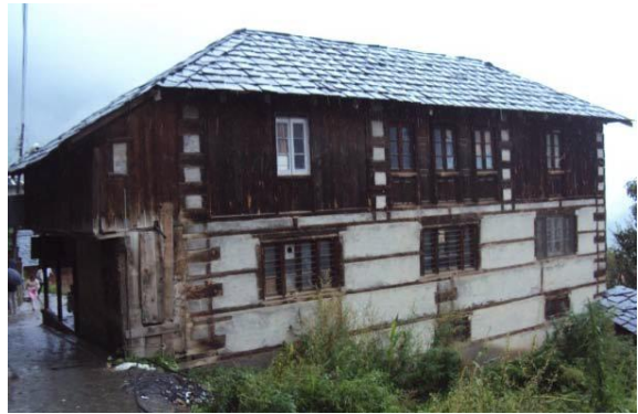
Figure 24: Wooden planks as infill in the upper storey - village Bharmour, Distt. Chamba (H.P.)
