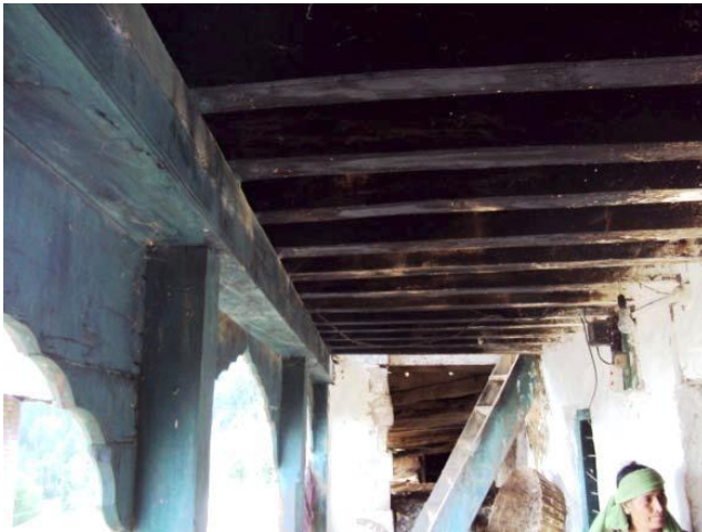
Figure 27: Main beam supported over posts (khambe) in the verandah and secondary beams also laid over main beam
