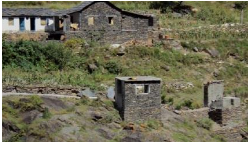
Figure 12: Typical Dry Stone construction
