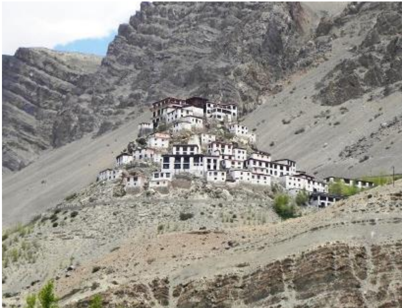
Figure 11: Typical Mud construction
