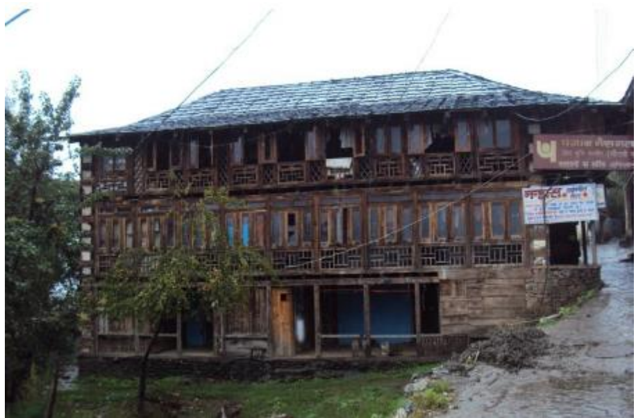
Figure 10: Typical Thathara house
