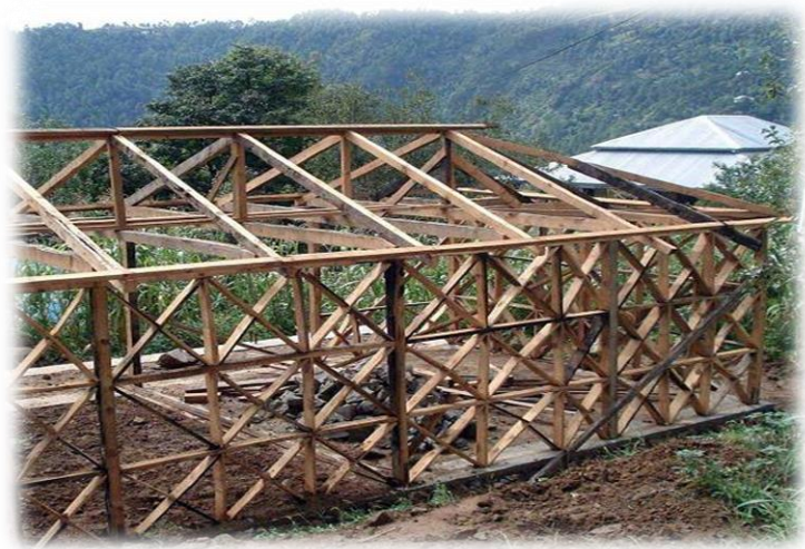
Figure 15: Typical Dhajji dewari framing
