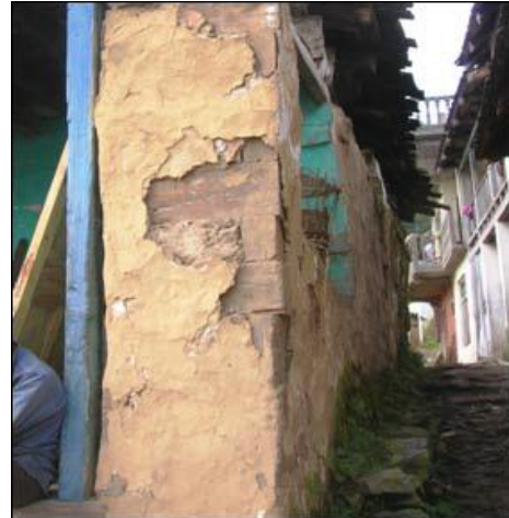
Figure 23: A mud plastered thathara
