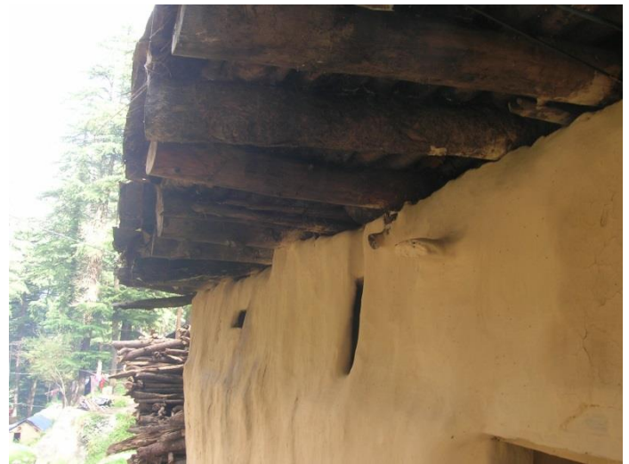
Figure 61: Connection between a flat roof and wall
