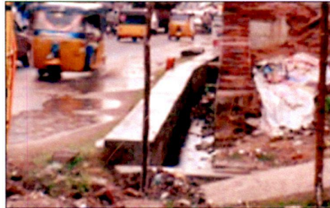
Fig 4.22:- Construction debris in drain
