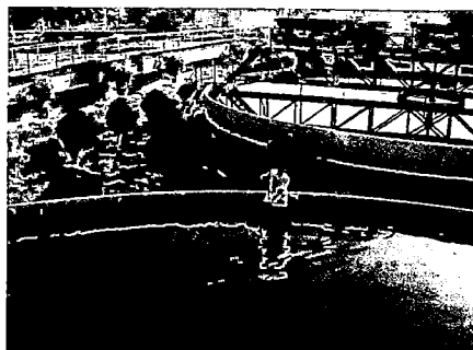
Figure 4.2.2: Secondary Settling Tank
