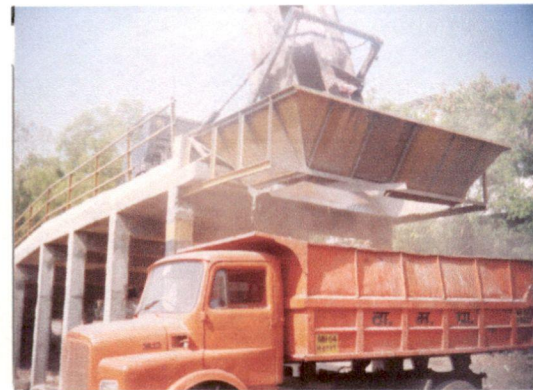
Figure 6.6 : Waste is being transferred from dumper placer to transfer vehicle
