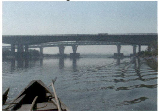
Figure 4.14: Shorter span Saket bridge behind longer span highway bridge
