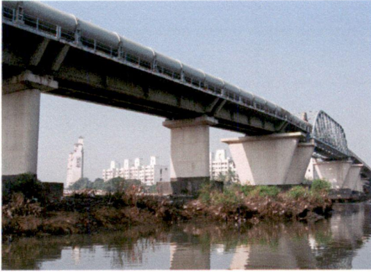
Figure 4.11: Blocked water way below 100 MLD Saket bridge
