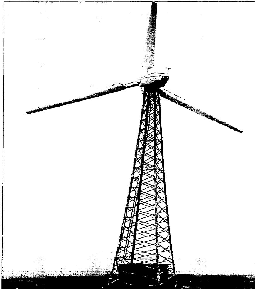
Fig. 3.6 A figure showing typical lattice type tower and nacelle (at Vijaydurg - Girye wind farm)
