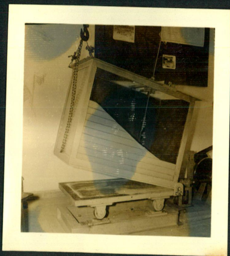
2. Tank shown in inclined position for the static test.
