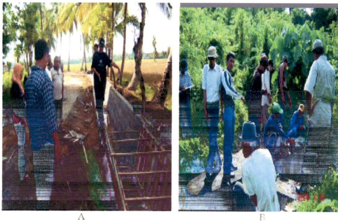
Figure A: Technical assistance in constructing MRC canal lining.
