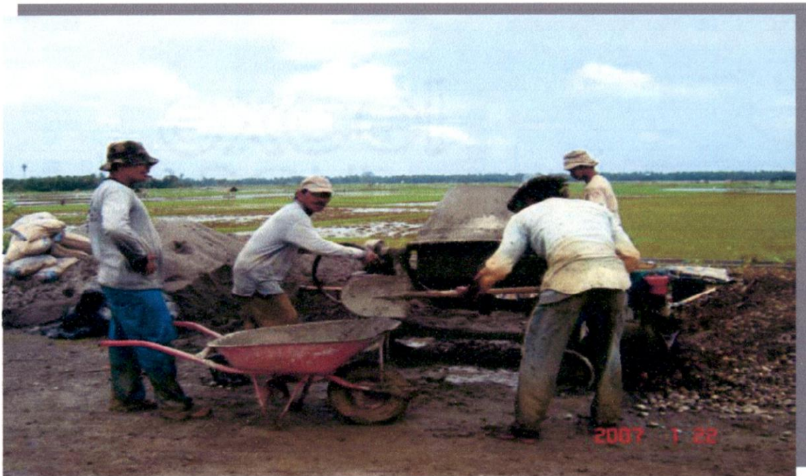
Figure A: Four WUA's members in Krueng Aceh Irrigation, Aceh Besar is "gotong royong" using a concrete mixer to prepare required materials needed to complete construction of tertiary canals.
